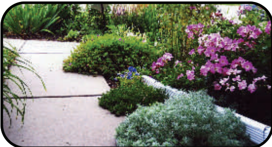
A downspout directing water to a garden.
