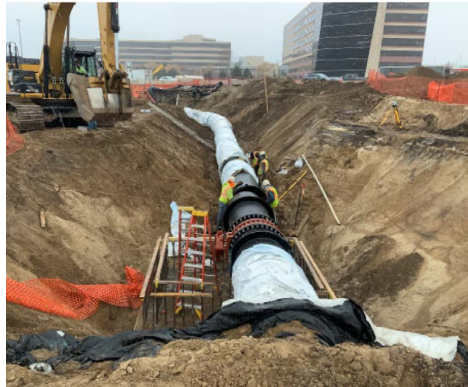
Construction crew installing the new 42" looking north from the south side of 494.
