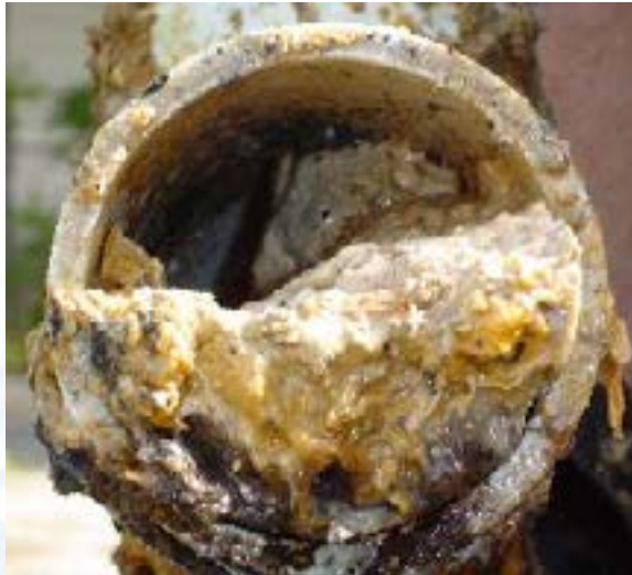
Blocked wastewater pipe.
