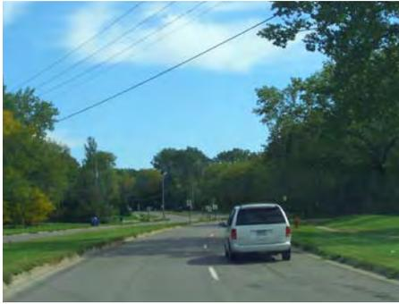
East of France on 90th Street, a median is provided along with a 4-lane configuration. Reducing this segment to a 2-lane plus turning lanes in the median effectively make this a 3-lane configuration with bike lanes on either side.
