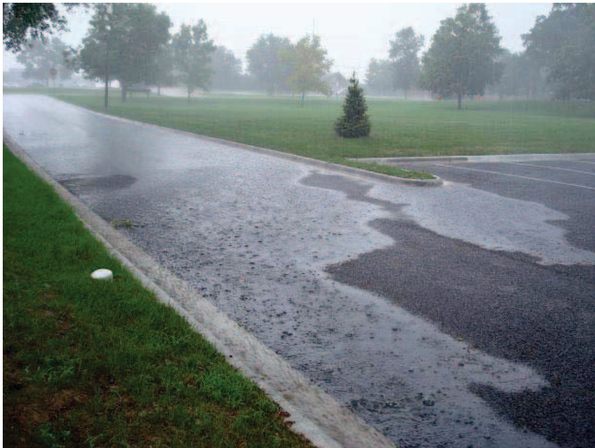
Impervious access driveway onto pervious parking lot
