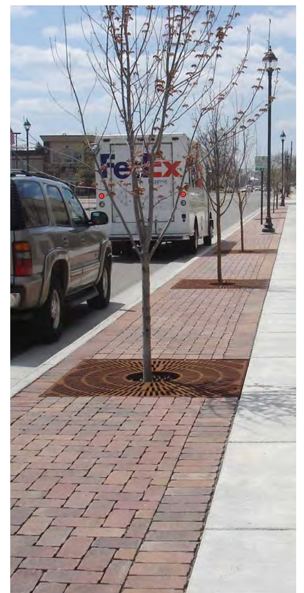
E. Tree trench using structural soils, permeable pavers, and tree grates
