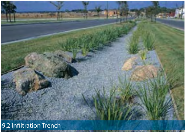
9.1 Infiltration Trench
