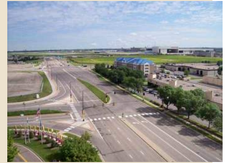
Aerial view of 24th Avenue looks north at Lindau Lane.
