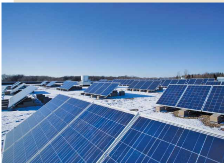
Photo voltaic panels provide active solar energy generation.
