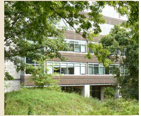
Ceridian is a good example of sensitive site and landscape design adjacent to the bluff.
