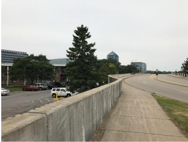
Bridge looking west over Normandale Boulevard.
