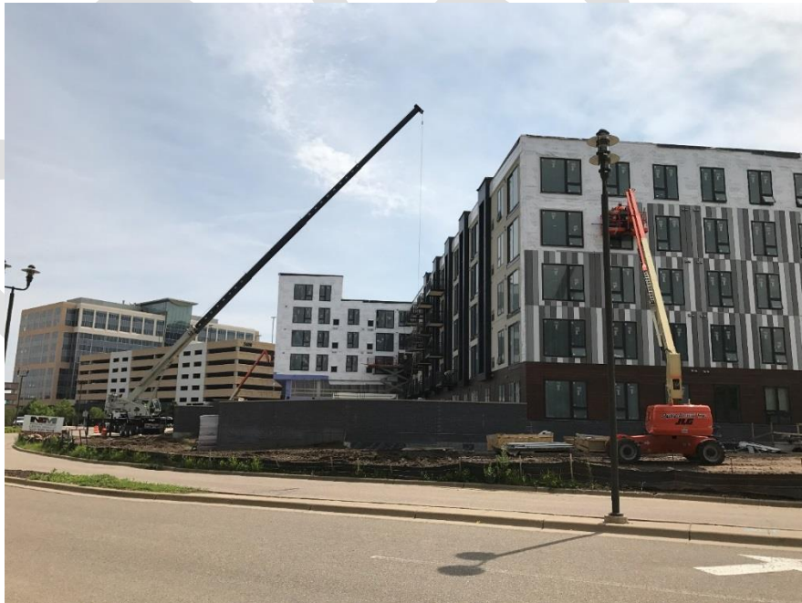
A 179 unit apartment building that is under construction.
