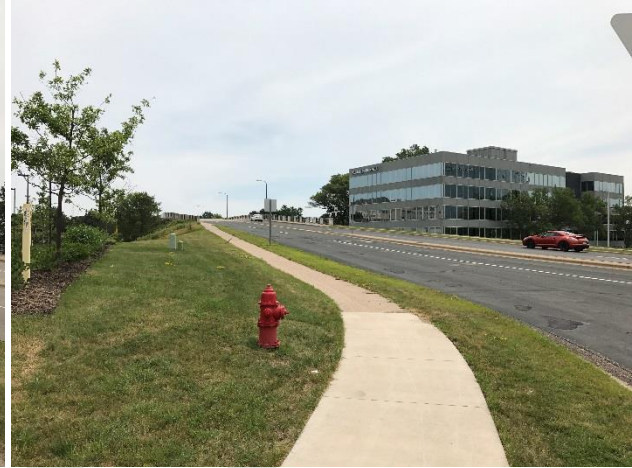
Bridge looking east over Normandale Boulevard
