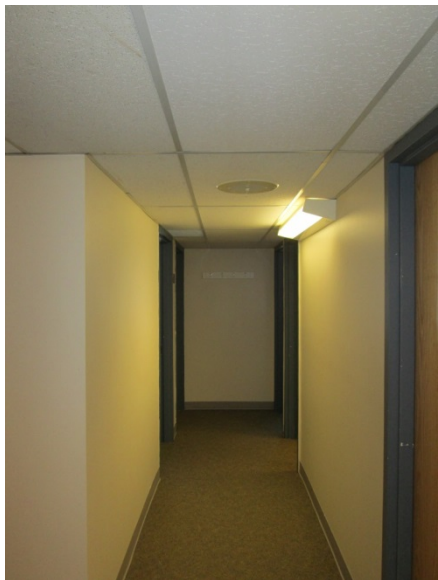
A few areas have lay-in ceilings of acoustic ceiling tile (ACT).
