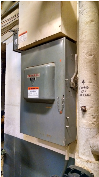
Main disconnect switch in the boiler room.
