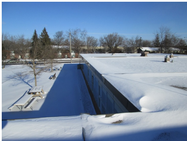
Better insulation and tapering is recommended with roof replacement.
