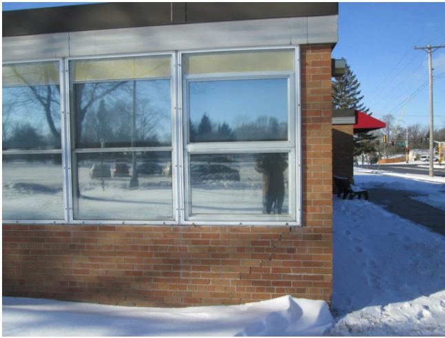
Repair and repointing mortar joints is recommended.
