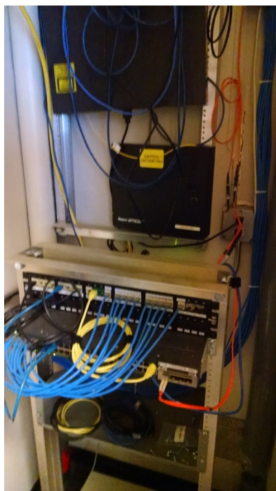
Wall mounted IT equipment without separate cooling system.
