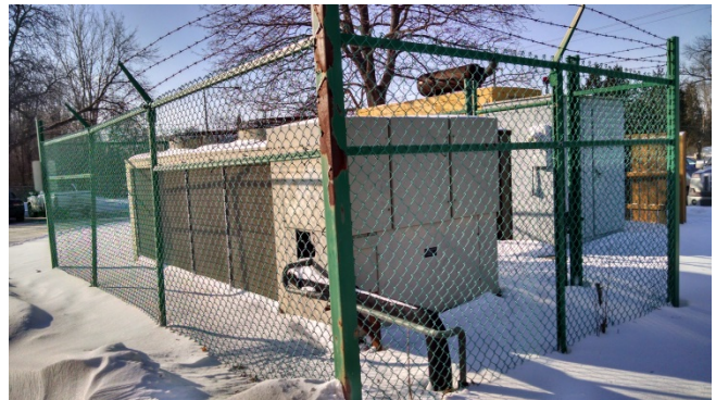
The chiller is tapped off the Xcel service and is not backed up by the generator.
