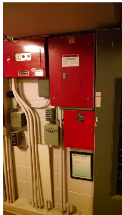
Existing Honeywell fire alarm system is not code compliant.
