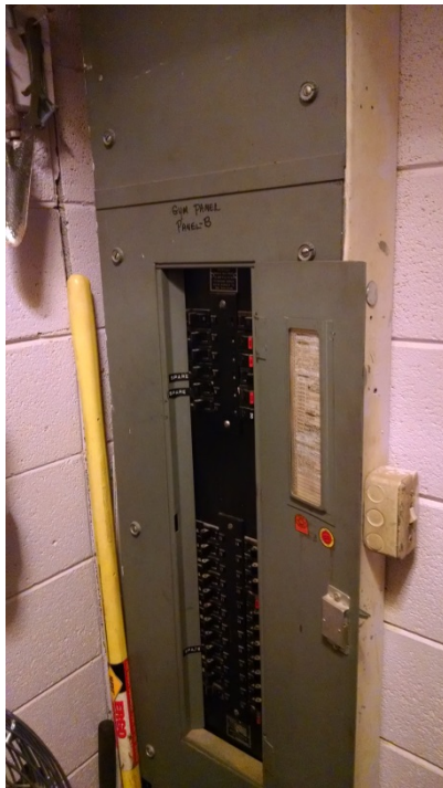
Original FPE brand electrical service equipment.
