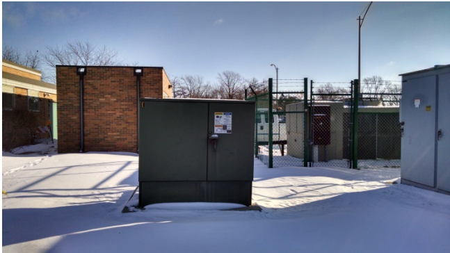
Xcel pad mounted transformer (225 kVA) outside the east wall of the building.
