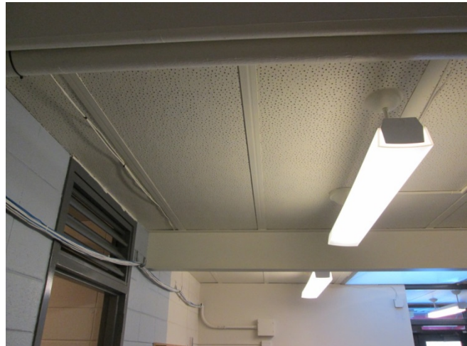
Acoustic form board ceiling is part of original roof deck construction.
