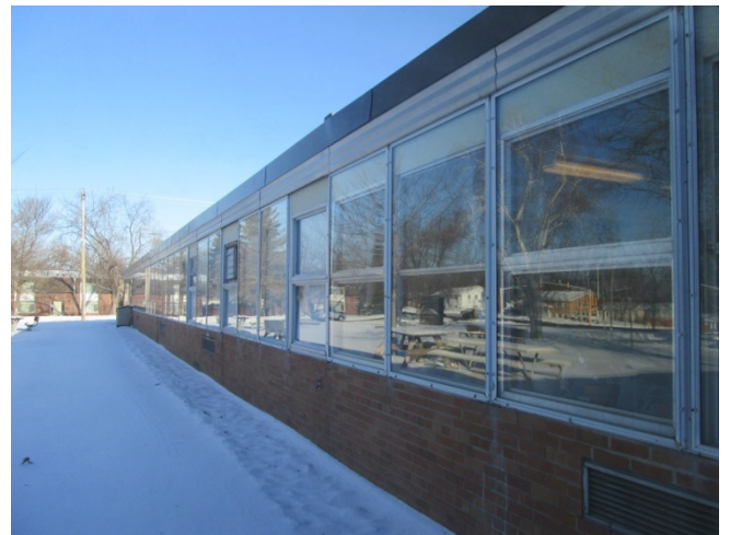
Glazed storm panels cover most original single glazed windows.
