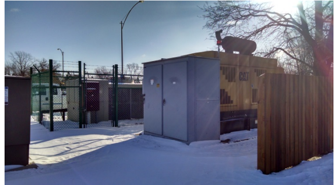
Transfer switch mounted at the emergency generator.
