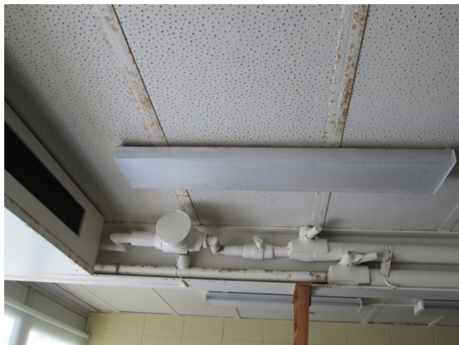
Evidence of moisture problems is visible.
