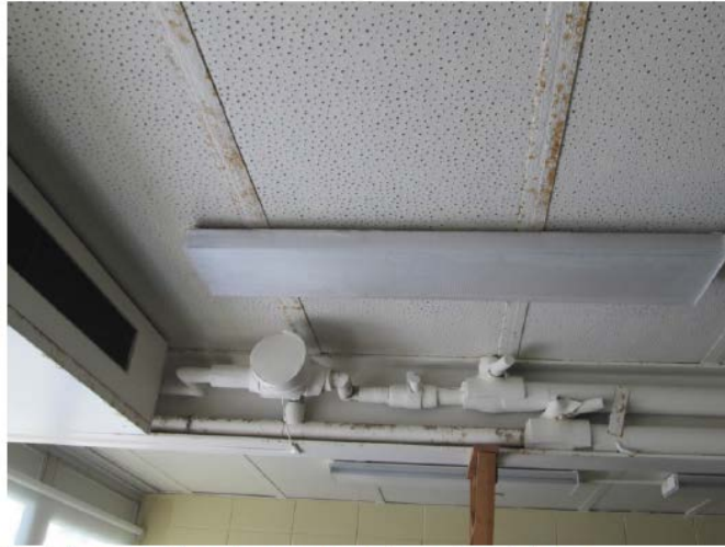
Evidence of moisture problems is visible.
