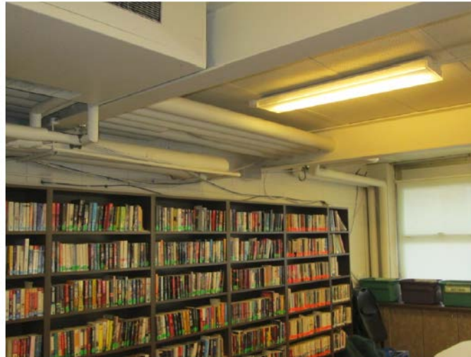
Low ceilings and exposed mechanical and electrical systems contribute to inflexibility of spaces.
