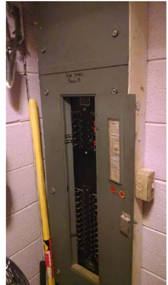
Original FPE brand electrical service equipment.
