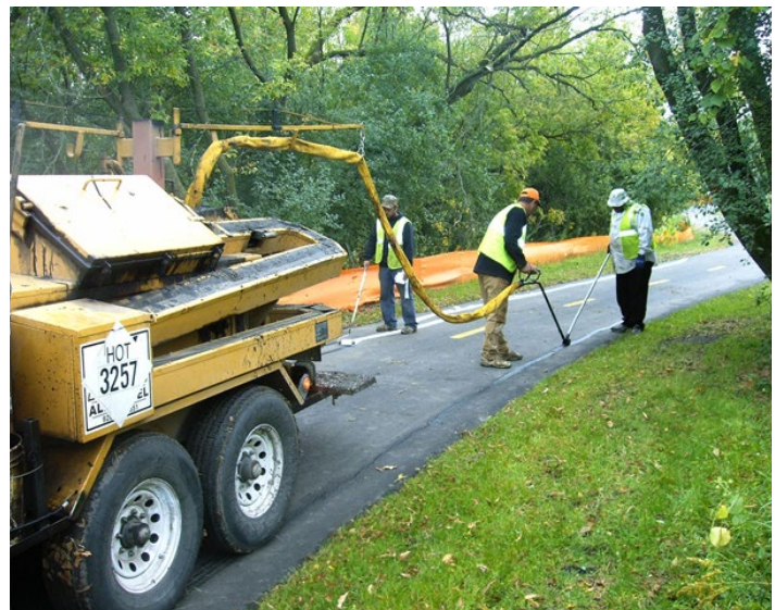
Asphalt crack repair and seal combined
