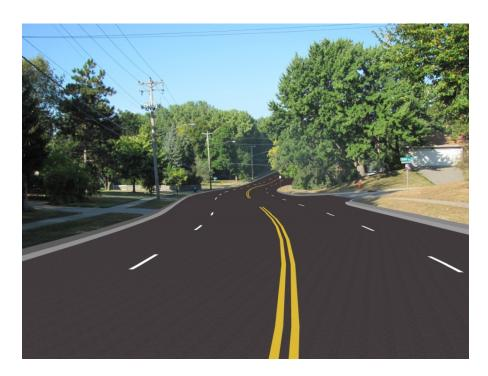
• Three-Lane Roadway – this option maintains the existing roadway width of 44 feet. It will be striped to include two 11-foot travel lanes, a 12-foot center left-turn lane and two five-foot shoulders. The existing on-street parking (time restricted) will be eliminated.
