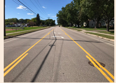
Conversion of 4-lane road to 3-lane road with bike lanes in shoulder.
