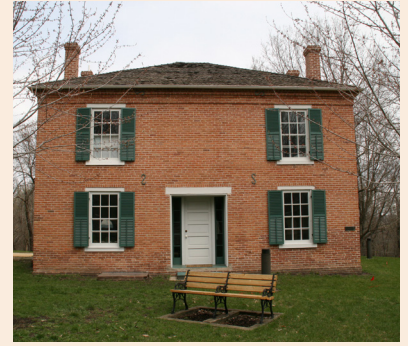
Gideon Pond House - a class 1 historic site.
