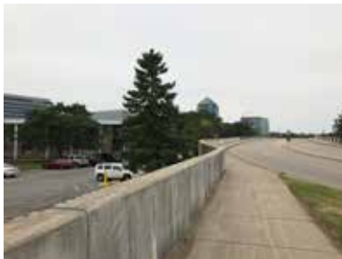
Bridge looking west over Normandale Boulevard.
