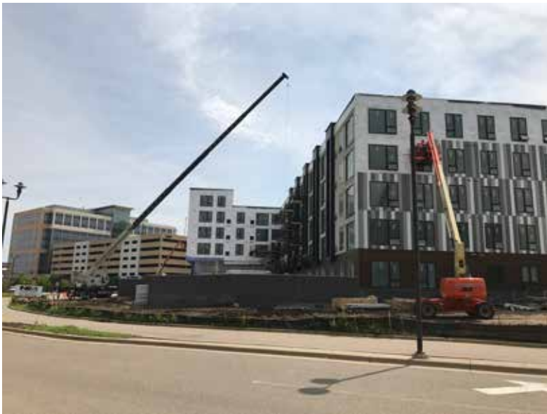
A 179 unit apartment building under construction.
