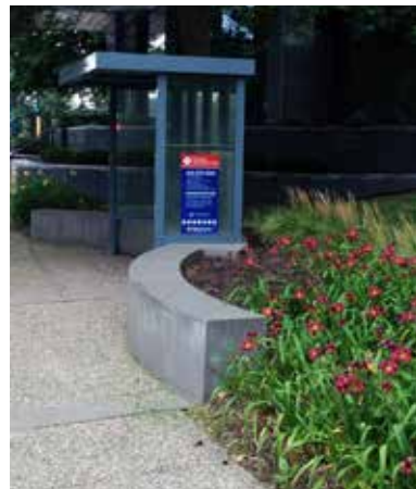
Enhanced bus stop with shelter.
