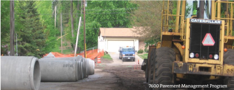
7600 Pavement Management Program
