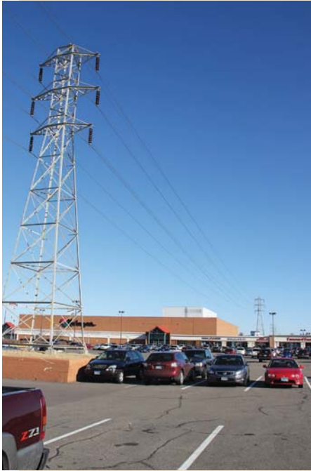
Overhead transmission line extends through Southtown Shopping Center site.
