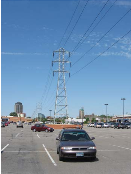
Existing electric transmission line
