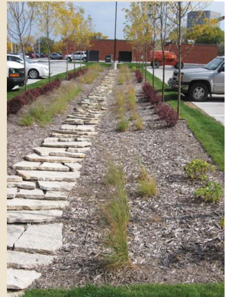
Bioswale in parking lot at Genesee Apartments
