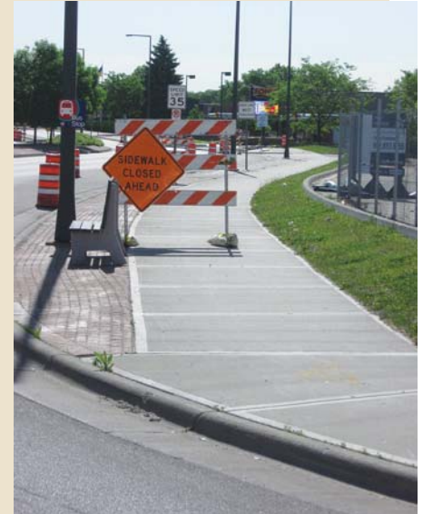
On going road and sidewalk improvements.
