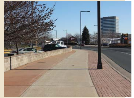
American Boulevard Core Pedestrian Way uses colored and textured concrete to enhance pedestrian experience.
