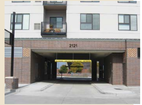
Access to parking located behind the building.
