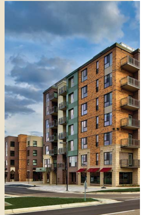
Genesee development at the southeast corner of Penn Avenue South and American Boulevard.
