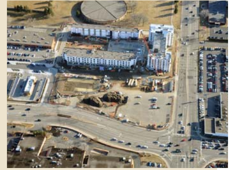
New mixed use development under construction in the District.
