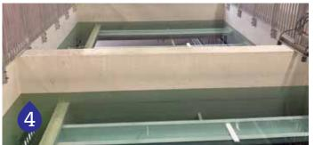
The water is filtered to remove any remaining particles, then enters an underground reservoir called a clearwell where small quantities of fluoride are added. Because fluoride promotes strong teeth and bones, fluoridation is mandated by state law at a dosage between 0.5 and 0.9 parts per million. See page WQR 4.
