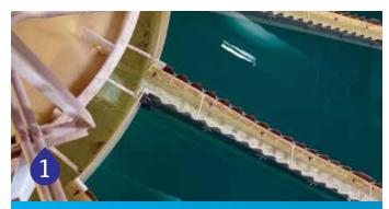
The softening process begins when slaked quicklime is mixed with raw water in one of the City's two solids contact basins. Each basin holds half a million gallons of water.
