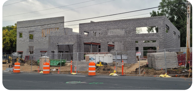
Construction of Fire Station #4, 4201 West 84th Street, September 2022.
