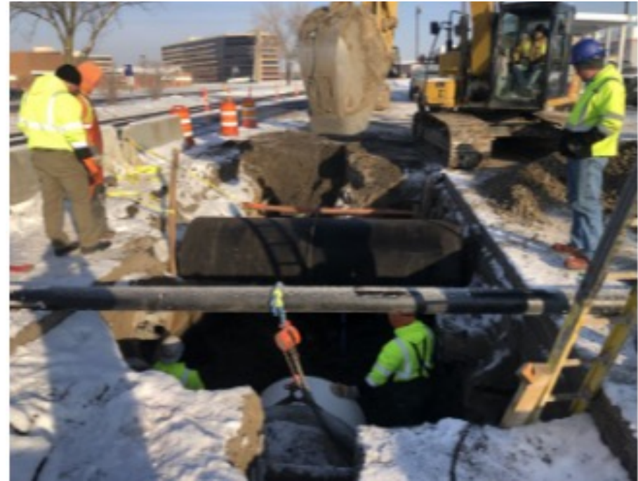
Photos courtesy Valley Rich Co. Inc. Photo on the top of repair pipe lowered into the hole; bottom photo after repair completed.
