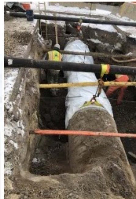
Photos courtesy Valley Rich Co. Inc. Photo on the top of repair pipe lowered into the hole; bottom photo after repair completed.
