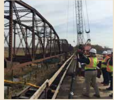
The Old Cedar Avenue Bridge is undergoing rehabilitation
