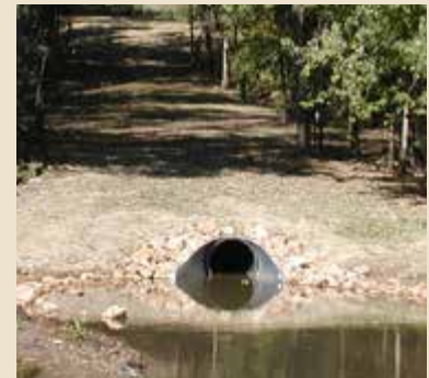
Storm sewer improvements at Mounds Spring Park
