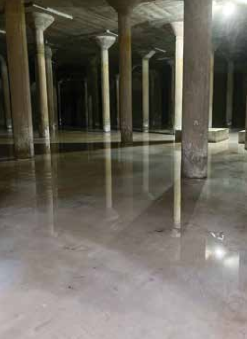
A dive inspection and cleaning project was completed on the City’s four-million-gallon clearwell (an underground storage reservoir) in 2020.
