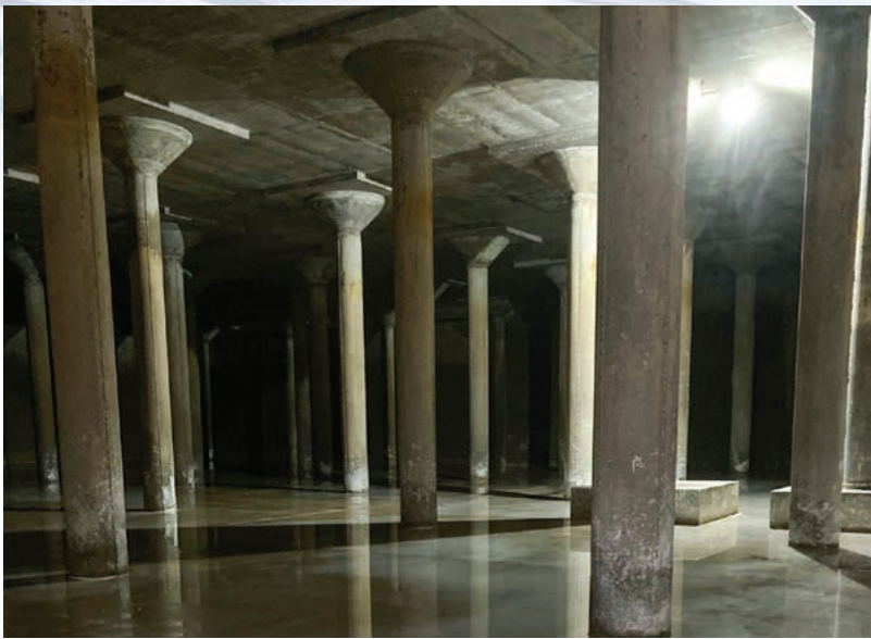
A dive inspection and cleaning project was completed on the City's four-million-gallon clearwell (final storage stage for water). While the clearwell is in excellent condition, a follow-up rehabilitation project is planned. Ongoing maintenance helps Bloomington water to consistently surpass state and federal requirements.
