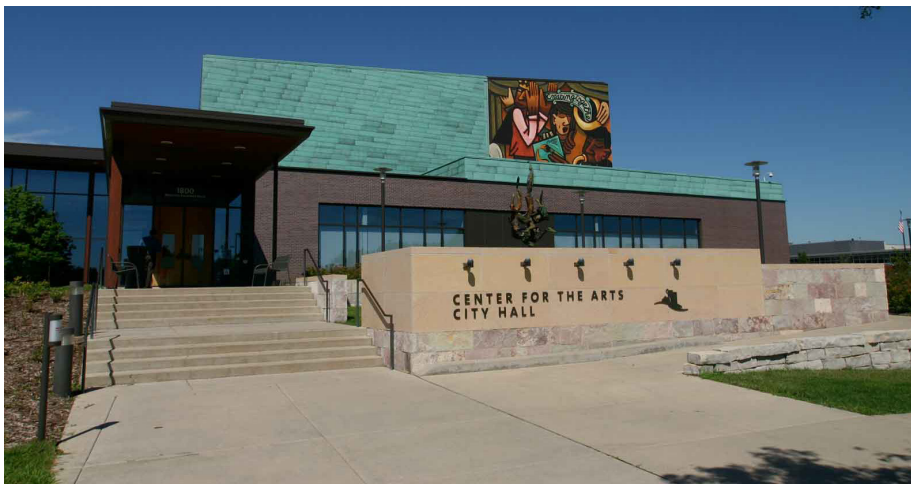
Center for the Arts at Bloomington Civic Plaza. Image courtesy of City of Bloomington and Creative Placemaking in South Loop.
