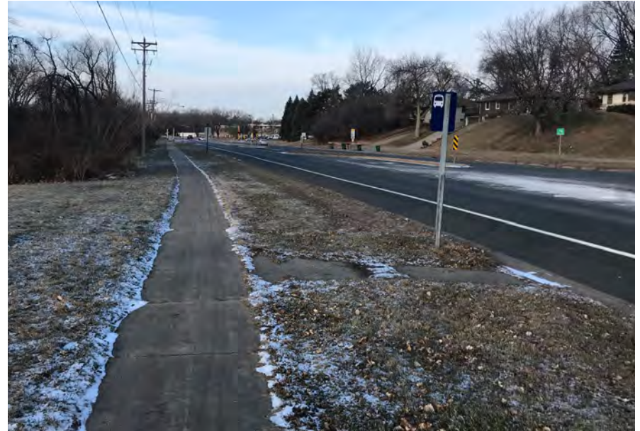
Narrow existing sidewalks - approx. 4' wide
