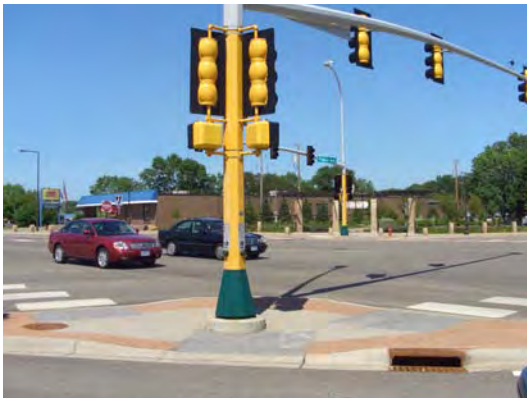
Raised medians, which are commonly used in Bloomington’s newer road designs adjacent to right turn lanes, provide refuge for pedestrians making longer street crossings.
