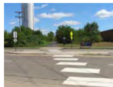
MN MUTCD standards are recommended for all roadway crossings to ensure consistency across the state.
