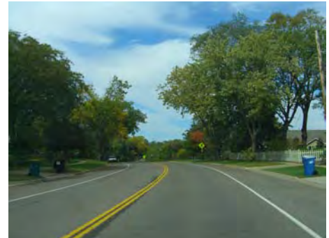
On the southern end of the Overlook Drive/Penn Avenue segment, a 2-lane configuration already exists, which is optimal for the entire corridor.
