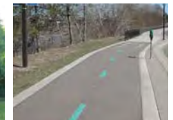
In some systems, a green center line is used in lieu of yellow as an identifier of a system of trails. If this approach is taken, maintain consistency to avoid confusion.
