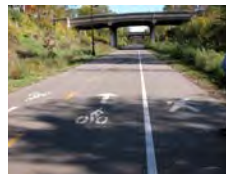
A solid white line may be used on a shared-use path to separate uses, with a broken yellow line used for separating opposing lanes. Pavement markings clarify proper uses and directions.
