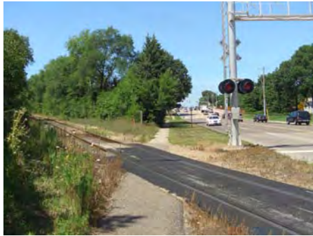
As this photo illustrates, three surfaces are used in one short segment. This lack of consistency diminishes the appeal of the corridor to pedestrians and bicyclists.
