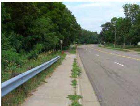
As this photo illustrates, the sidewalks vary in width and location, reducing a pedestrian's desire to walk along this segment. Being directly adjacent to the road also introduces concerns about separation from vehicles.
