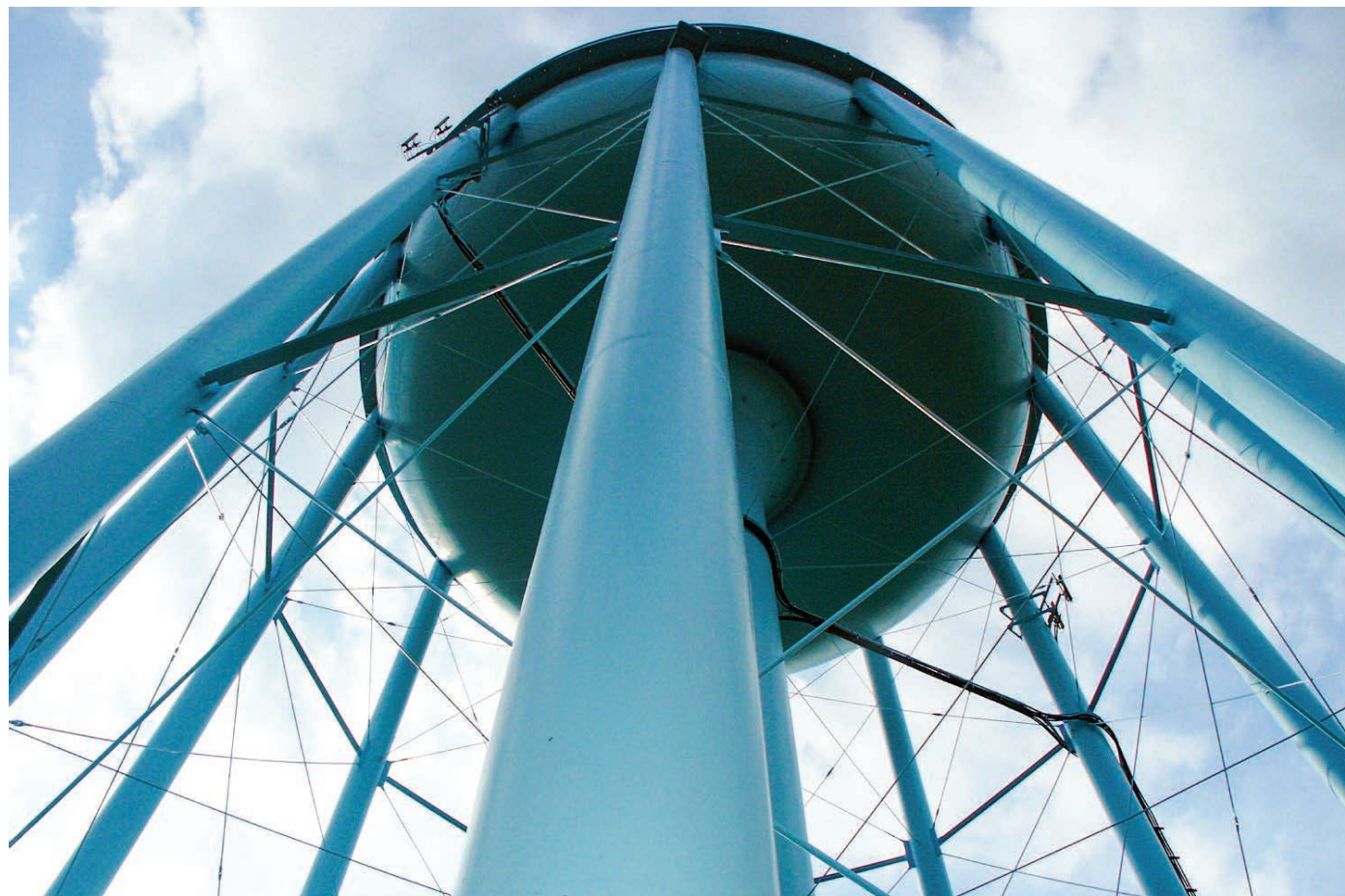
Bloomington's six water storage facilities provide the storage and maintain pressure that helps to keep drinking water flowing.
